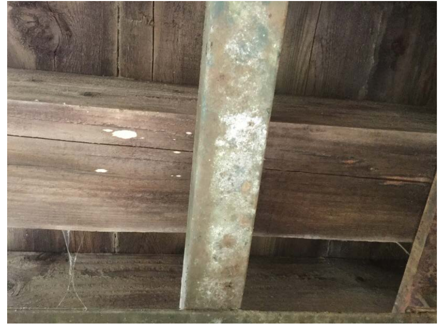
Timber deck from underneath
