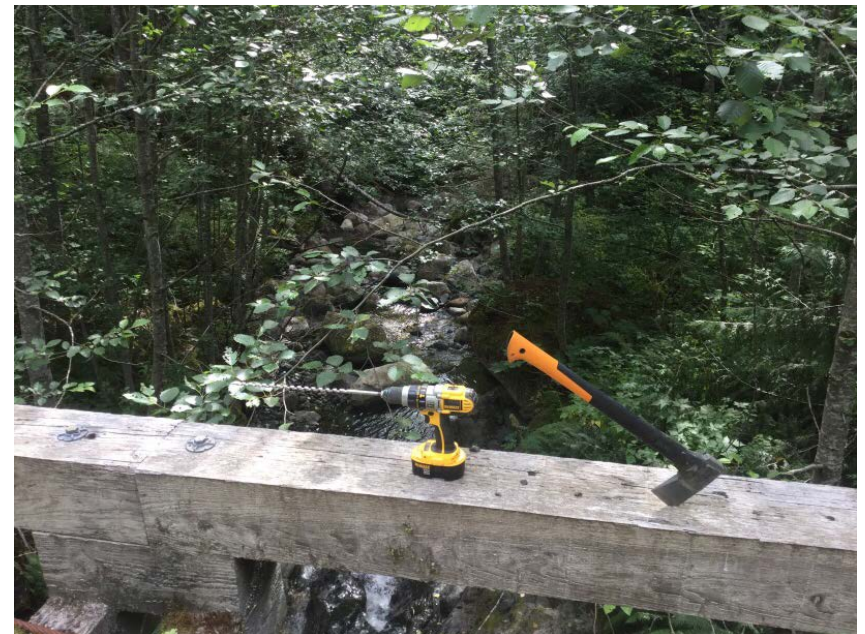
Looking downstream from deck
