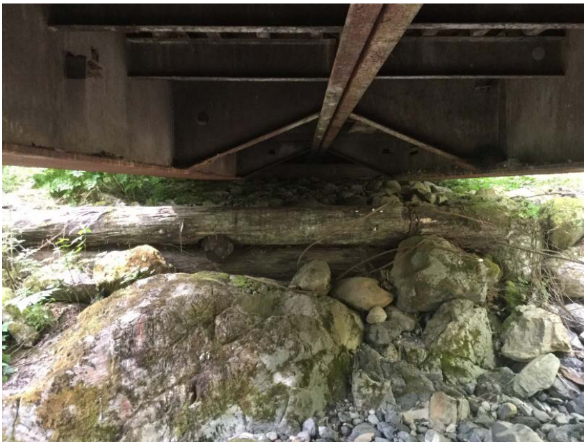
Right Bank Abutment when facing downstream
